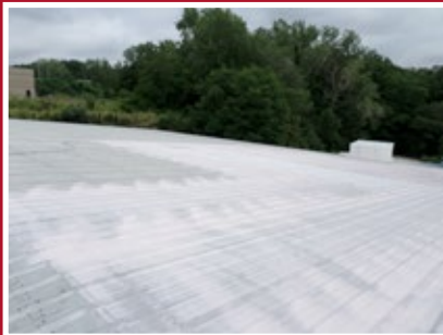
Roof primed with GacoFlex E5320 2-Part Epoxy Primer.
