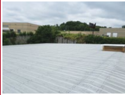
Roof after prepping and power washing.
