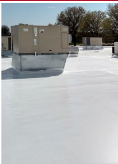
After the roof restoration was complete.
