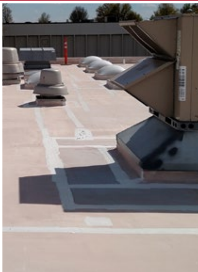
GacoFlex E5320 2-Part Epoxy Primer/Filler and GacoFlex SF2000 SeamSeal applied before GacoFlex S20.
