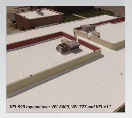
VFI-3600 Polyurethane Basecoat is a two component, aromatic polyurethane coating that forms a tough elastomeric membrane, that provides waterproofing and impact resistance when applied to the existing roof substrate.
