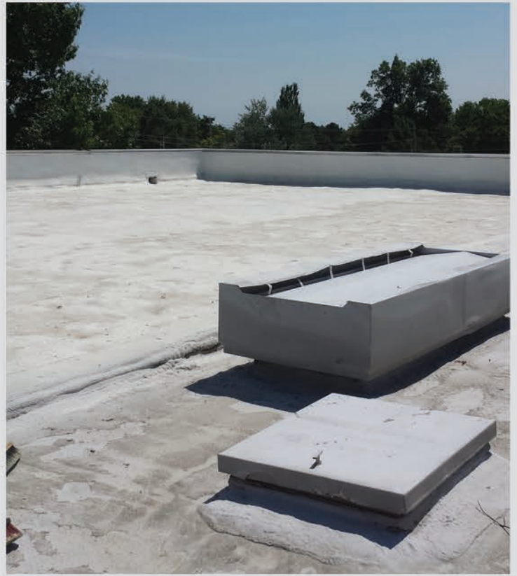
Before VFI-727 Polyurethane Foam and SEALGUARD VFI-990 SILICONE
